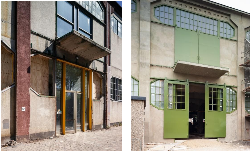
The south façade of Fenix Warehouse II, before and after restoration. Photos: Rubén Dario Kleimeer
