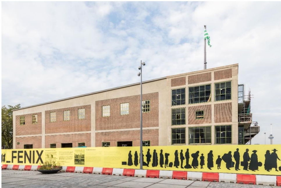
The eastern façade of the Fenix Warehouse II after restoration, photo: Sylvana Lansu
